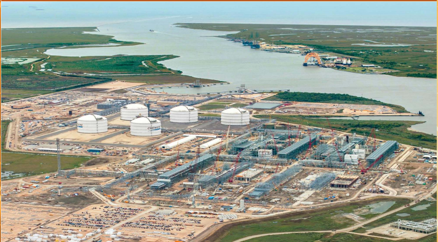
Cheniere's Sabine Pass Project. Source: Cheniere
