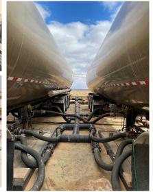
(Above) 45,000 bpd self contained High Spec treatment facility. Pulling produced water directly off a pipeline with the ability to divert back into a pipeline or storage pit to stack water for high demand frac use.
